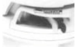
Flushing lever (black) and water fill lever (white) shown in the normal closed position.
